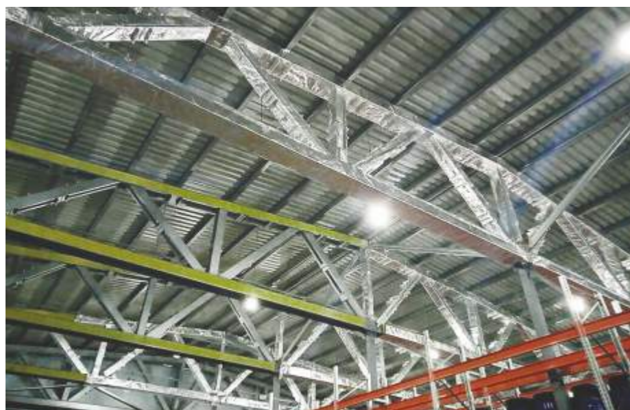
Protection of light steel thin-walled structures
